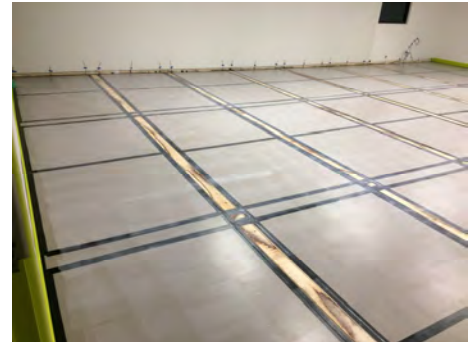
Figure 23: The heating panels installed
