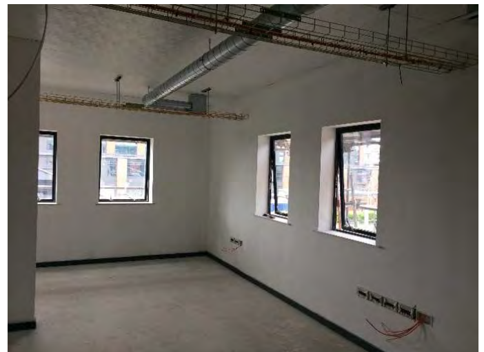
Figure 55: Internal view of first floor office
