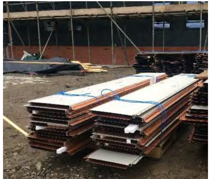
Figure 41: Cladding panels pre-installation
