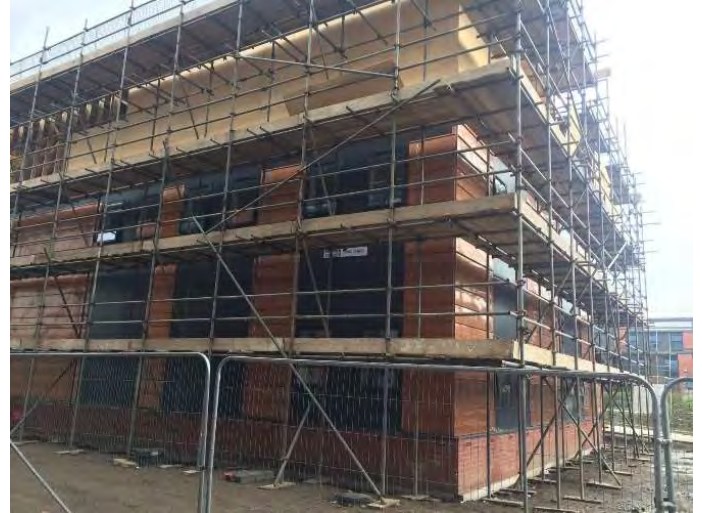
Figure 48: External cladding installation
