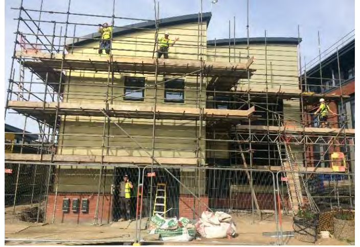
Figure 56: Seren Gold cladding on east elevation and living wall filling
