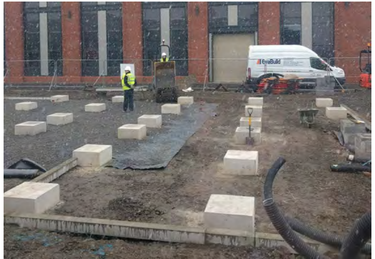
Figure 7: Concrete Pad Foundations
