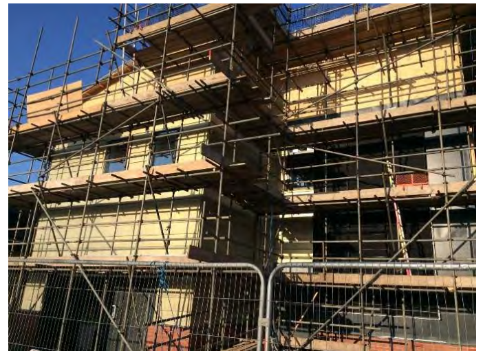
Figure 51: Cladding and living wall trough installation on east elevation
