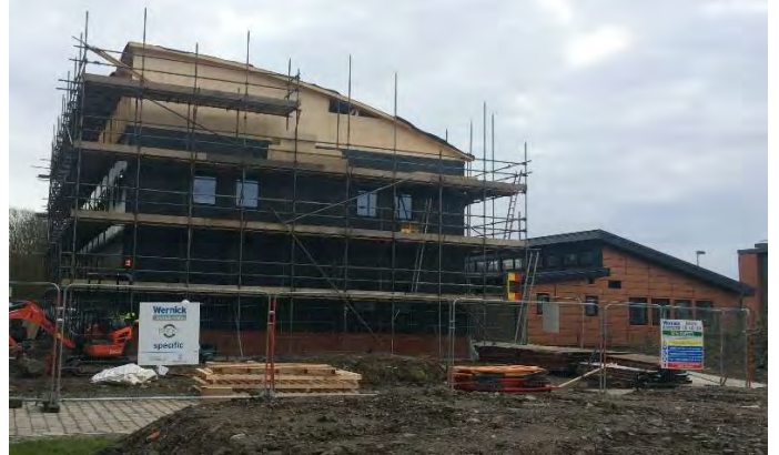
Figure 40: Roof construction – pre-cladding installation
