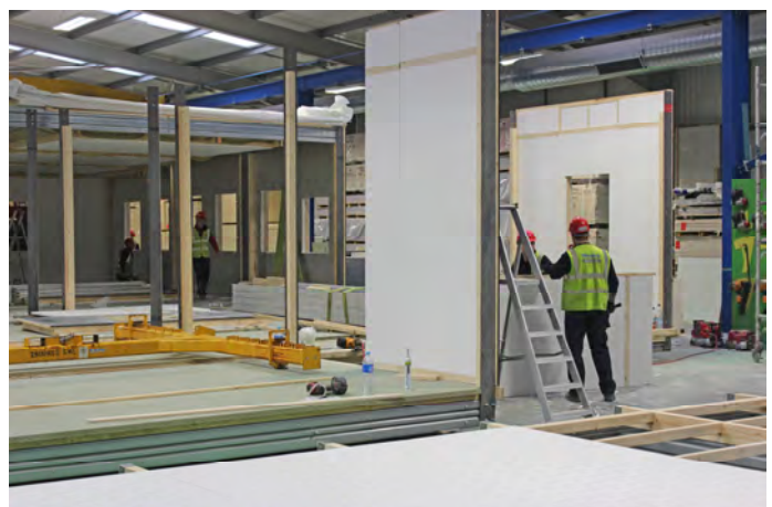
Figure 31: Module construction in the factory
