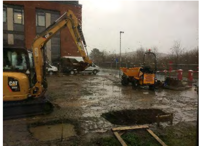
Figure 32: Site works commencing
