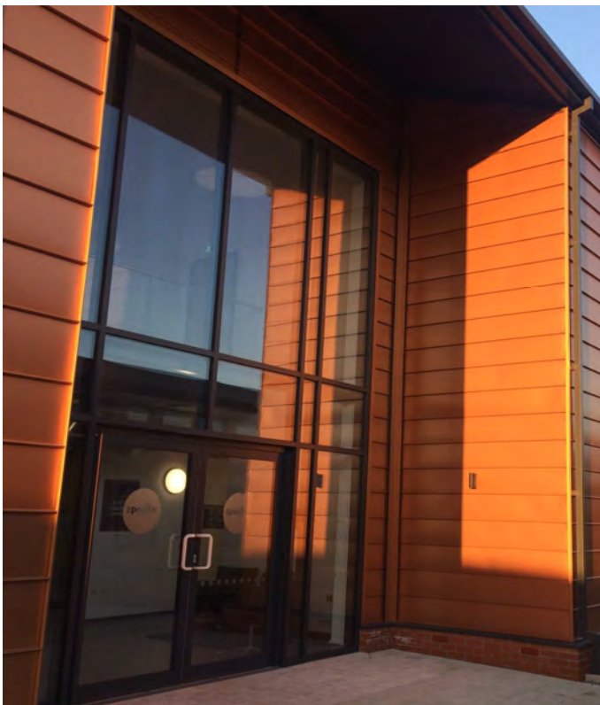
Figure 16: Curtain walling at main entrance
