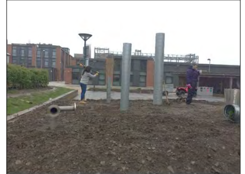
Construction waste re-utilised
