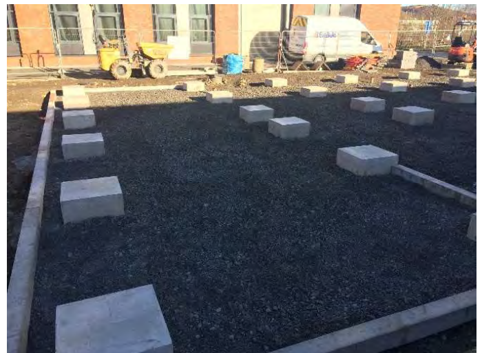
Figure 35: The concrete pad foundations
