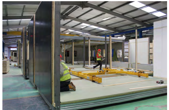
Figure 33: Module construction in the factory
