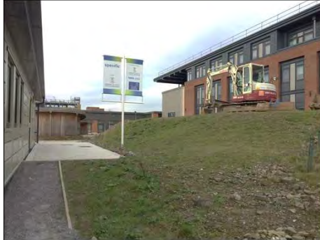
Excavated spoil redistributed on site
