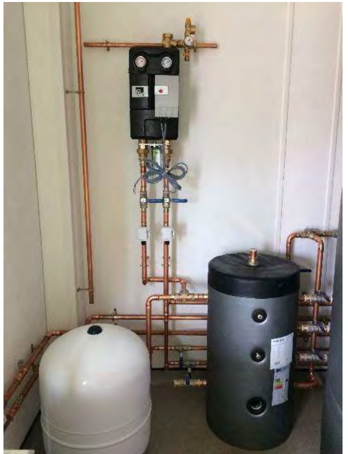
Figure 46: Heating system installation
