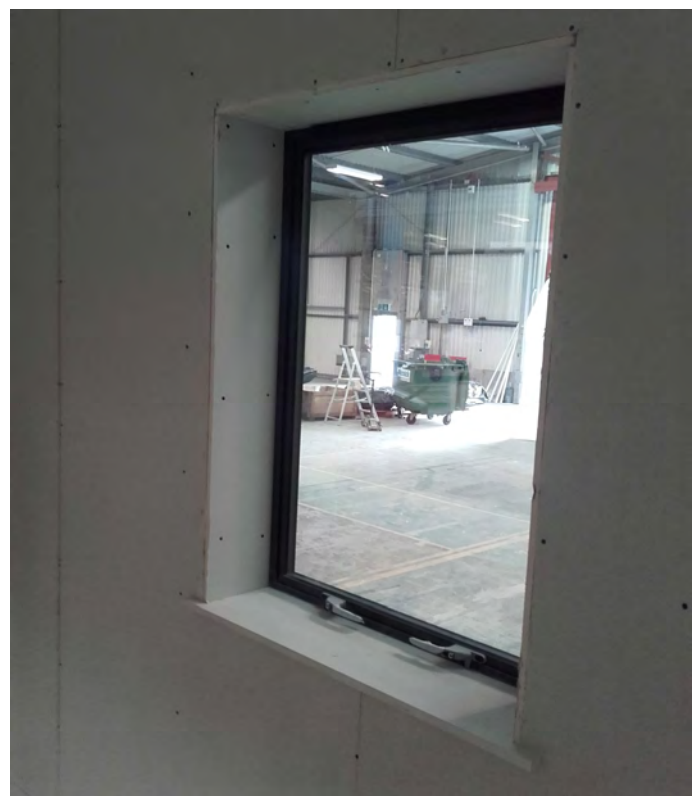
Figure 17: Window positioning within the external wall
