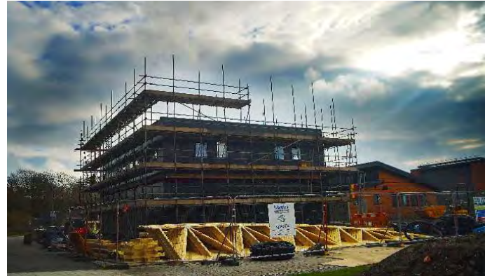
Figure 37: Scaffold erection
