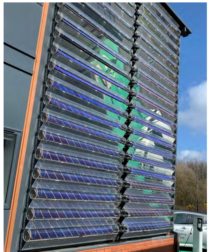
Figure 71: The PVT array in situ on the south elevation
