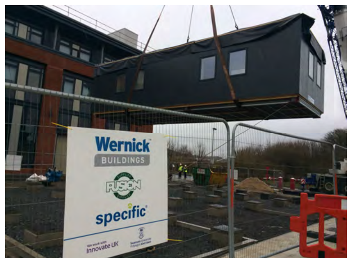
Figure 36: Modules arriving to site
