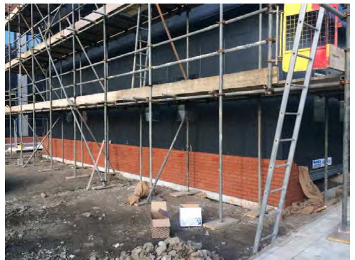
Figure 39: the brickwork plinth
