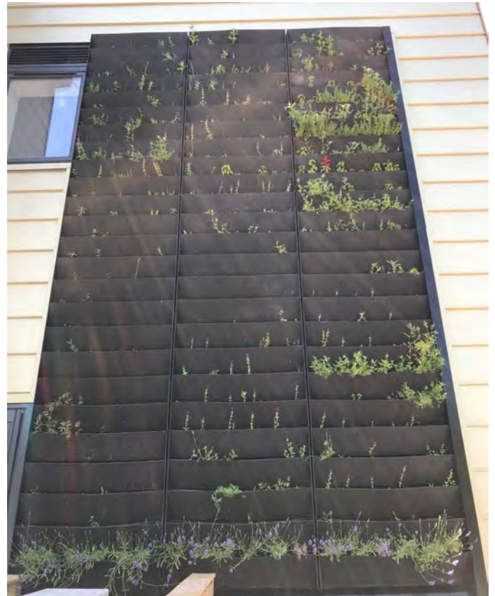
Figure 74: Living wall just after project completion
