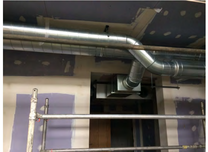
Figure 47: Internal decoration and M & E first fix
