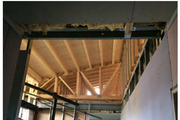
Figure 13: The glulam beams above the entrance foyer
