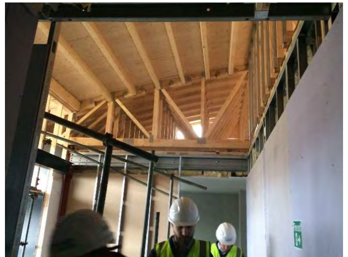
Figure 42: Roof construction above the entrance foyer
