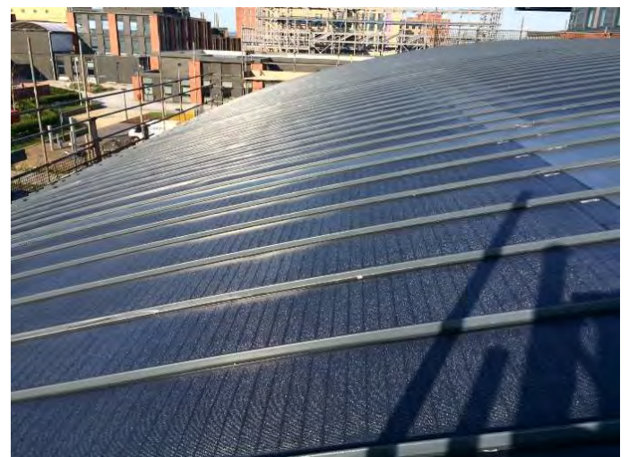
Figure 52: Completed curved BIPV roof
