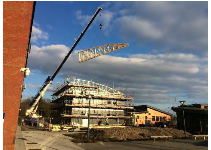
Figure 38: roof truss installation
