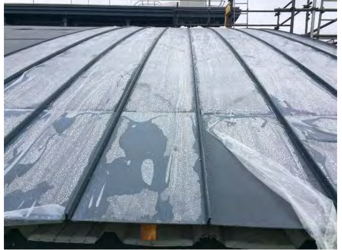
Figure 45: The BIPV roof installation
